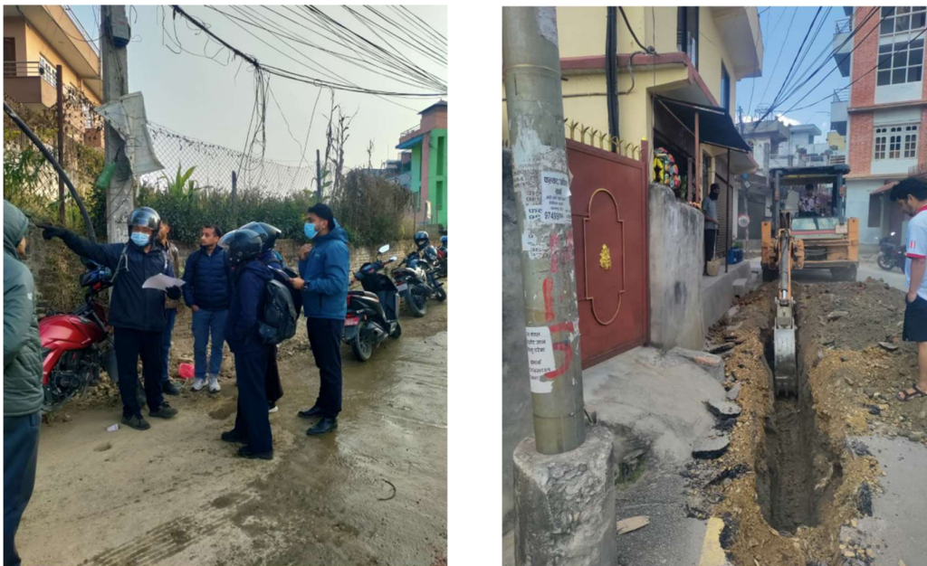
Node selection for valve installation
