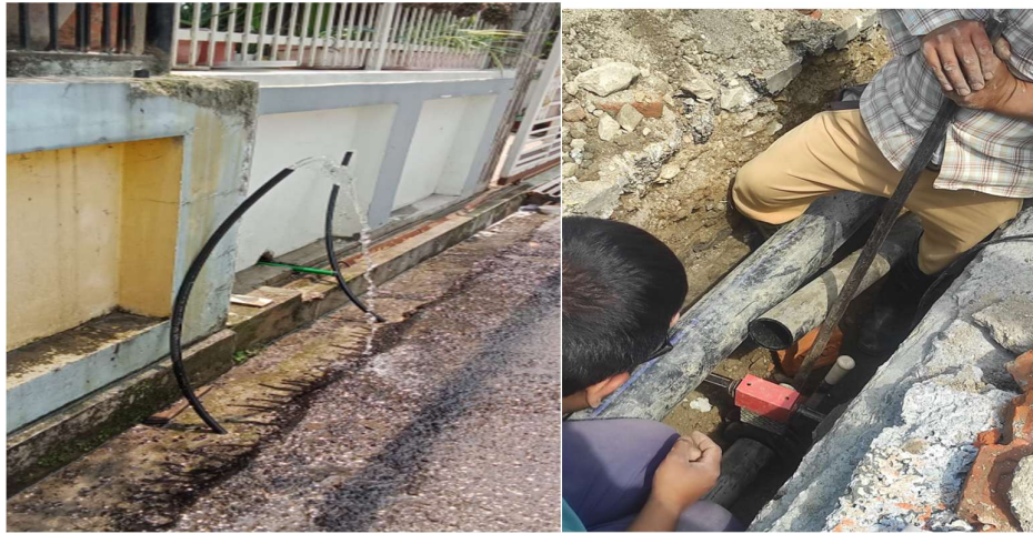
Pipeline मर्मत तथा water flow testing
