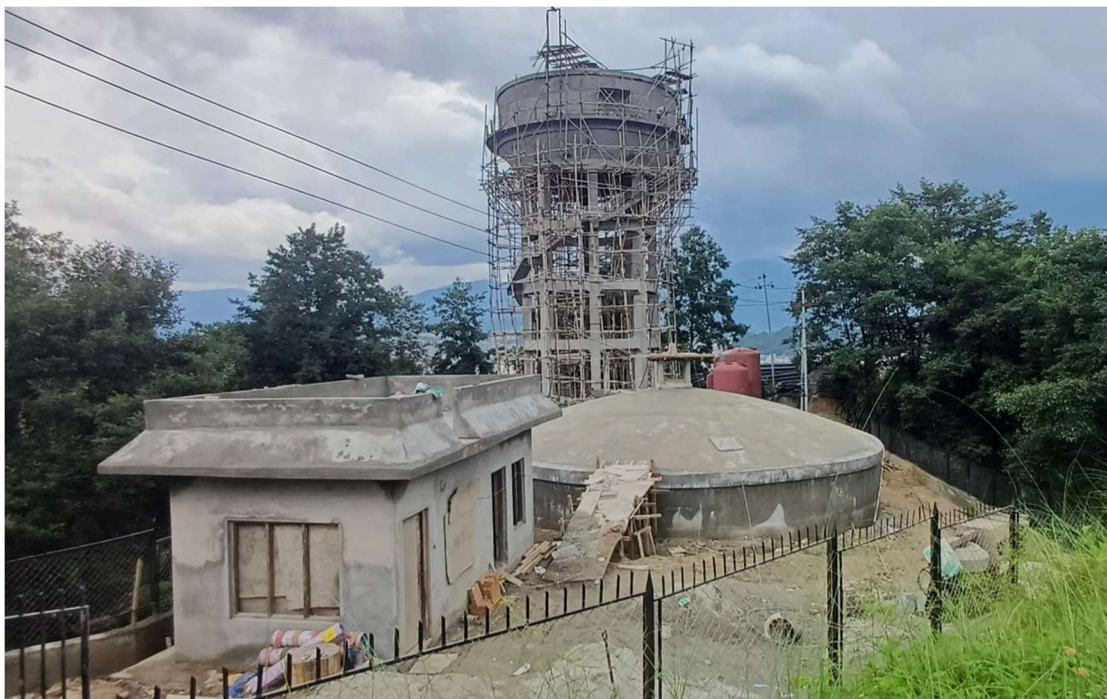
निर्माण सम्पन्न OT , underground guard house & filter plant
